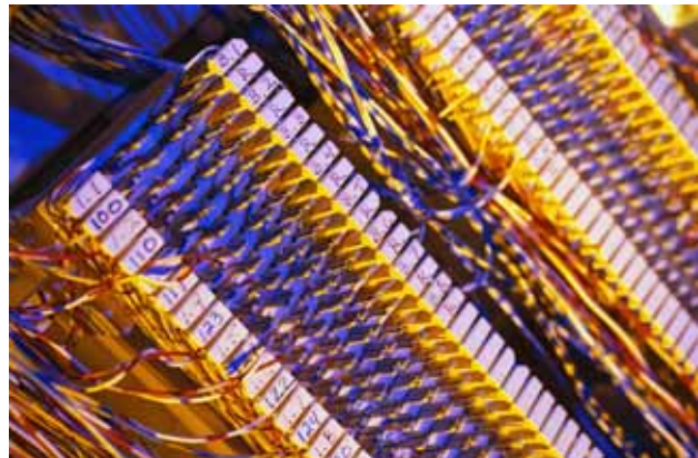
Figure 1.12 – Terminal Block
